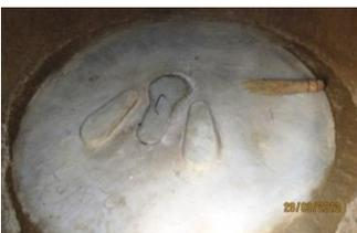
**Cement slab, installed level with earth floor around it**
