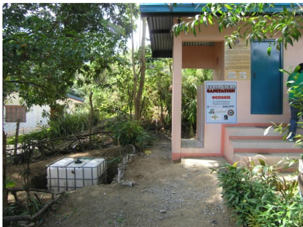
Figure 3. Simple collection container for urine using an IBC container. Example from the Philippines. Photo: Ebba af Petersens
