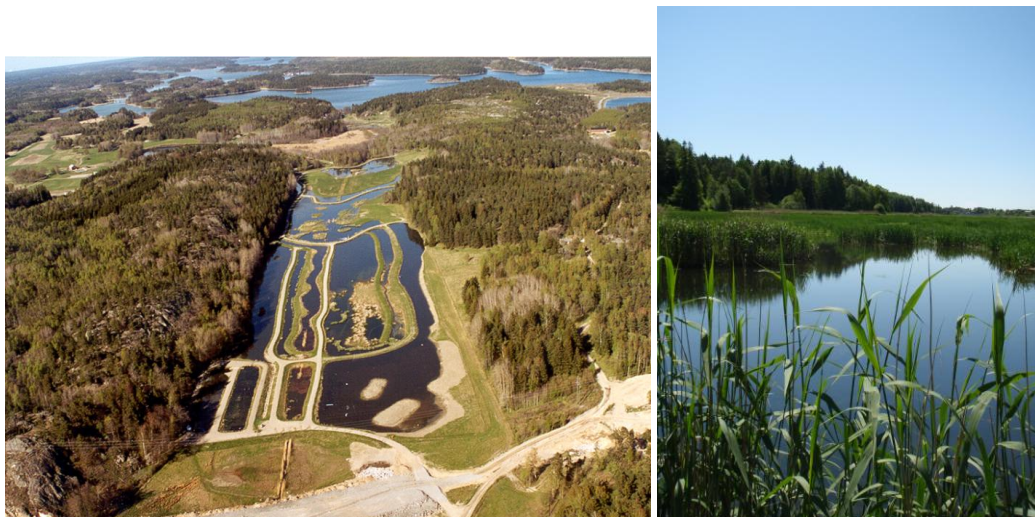
Figure 14. A constructed wetland for treatment of effluent from a wastewater treatment plant. The wetland acts as a biological step and reduce the content of bacteria and nutrients in the wastewater. Photos: Marcus Nilsson; WRS.
